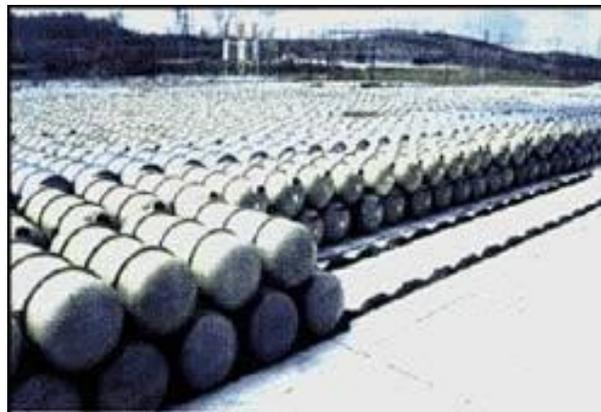
Figure 16. Concrete-floor storage yard for depleted uranium UF<sub>6</sub> cylinders at the Portsmouth, Ohio enrichment plant.
